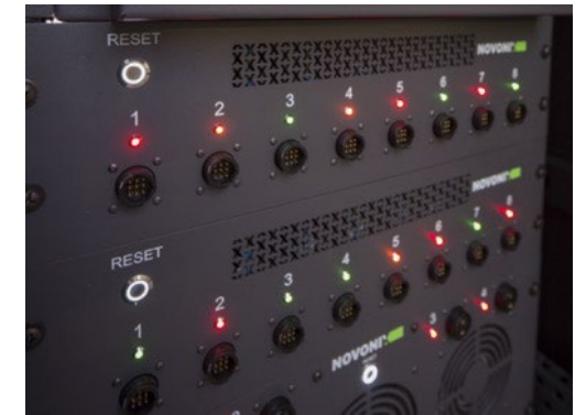
Diagnostic tools and performance testing
