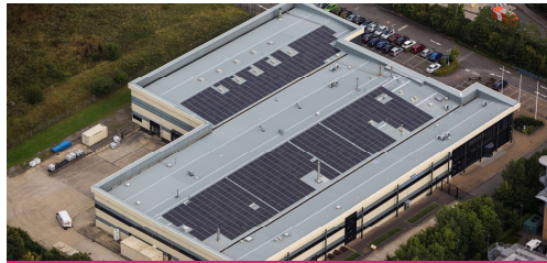
Industrialised and secure supply chain
